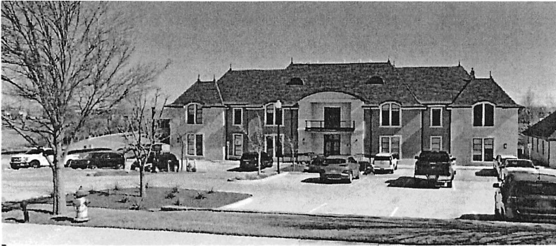
(Office building observed from Muirfield Place)
