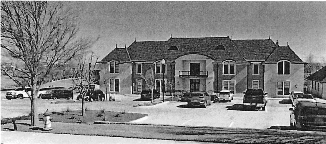
(Office building observed from Muirfield Place)
